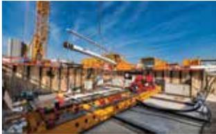
E-Power Pipe® is used for the trenchless installation of small-diameter product pipes at shallow depths. Over long distances of more than one kilometer, both pressure-resistant and non-pressure-resistant product pipes are installed quickly, safely and precisely. The two-stage process integrates aspects of the proven horizontal directional drilling (HDD) technology and pipe jacking (microtunnelling).
