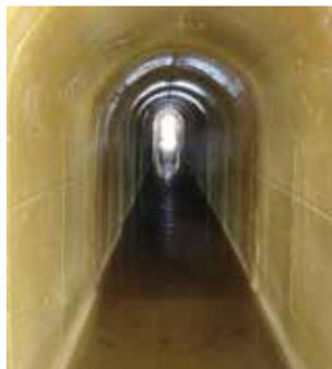
SprayWall is a self-priming polyurethane lining that reinstates structural integrity while providing infiltration control and chemical resistance. SprayWall's quick curing time allows the newly protected structure to be returned to service shortly after the application is completed,
