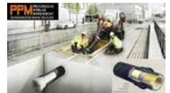
PPM technology utilizes a patented pressure drum to install, by means of inversion, a composite material liner in any metallic gas pipe. The liner is made of seamless circular woven fabric made of polyester yarns with a polyurethane non-permeable skin. Our product extends the life of the gas pipe by 100 years and has over \$12M invested in itesting by NYSEARCH/PHMSA and Cornell University.
