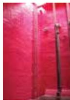
SpectraShield is a patented, polymeric lining system designed to stop infiltration and prevent corrosion in wastewater structures. A
