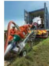
THE SHOOTER® is the original continuous air-inversion machine for CIPP and for decades has been a standard in the trenchless
