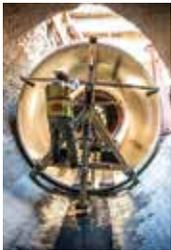
HOBAS pipe is suitable for virtually every installation method of new construction and rehab. The centrifugally cast, fiber-reinforced, polymer mortar
