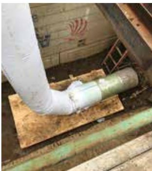
Aegion continues to advance the pipeline rehabilitation market by offering the latest innovations in cured-in-place pipe (CIPP) technology specifically engineered for drinking water applications. The InsituMain™ System, our showcase CIPP innovation for pressure pipe renewal, is a composite material of polyester fiber, fiberglass, and a specially formulated epoxy resin system.
