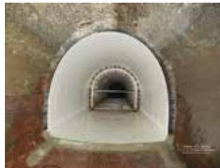
Danby PVC lining is a grout-in place structural solution for rehab, new construction and precast with H2S corrosion protection of pipes less than 36" and any shape/size structures. The Danby process is 100% trenchless using existing access/manholes, no proprietary installation machinery and no weld strips, and can navigate through curves and changes in shape or size.
