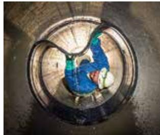
The WEKO-SEAL®, the industry's leading internal joint seal technology, is used extensively for internally resolving joint leakage, punctures and crack repairs in pipelines ranging in diameter from 18" and larger. Its unique design incorporates a series of proprietary lip seals that create a leak-proof fit on either side of the joint. With the WEKO-SEAL®, the leaks stop here!
