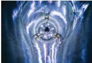
SAERTEX multiCom's UV-cured GRP lining products offer exceptional structural strength, resulting in thinner liners with increased hydraulic capabilities. Our liner technology offers optimal quality control with minimal equipment on site, minimal energy demand for curing, and reduced impact on the public. Applications include stormwater, wastewater, culverts and pressure pipes.
