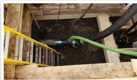
Abrasive airborne pipe cleaning
