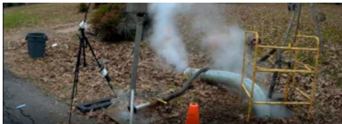
Figure 1. Emissions from an air cure CIPP Project
