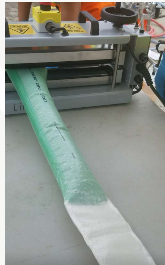
Wet-out liner before resin distribution and calibration
