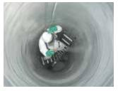
4553® Epoxy Coating is a specialty coating system for brick, block, concrete or fiberglass manholes; manholes with force-main discharges, deteriorated pipes, and wastewater treatment plant structures exposed to harsh chemical environments. The 4553® Epoxy Coating over Reliner MSP® Cement may be [hand] applied, mixed with aggregate, to get a quick 24-hour, abrasion-resistant, structural repair in critical structures.
