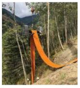
The Omega UV Liner is constructed with ECR (corrosion-resistant) fiberglass and advanced UV resins – proven to be one of the strongest on the market. Omega Liners are manufactured using unsaturated polyester or vinyl ester resins for environmentally conscious projects and are offered from 6" (150mm) to 66" (1675mm).
