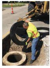
The Cretex PRO-RINGTM, a solid, lightweight, watertight alternative to concrete grade adjustment rings and brick & mortar used to adjust manholes, catch basins and utility structures. HS25-load-rated and passes ASTM C-1244 (vacuum test). Thicknesses from ¾" to 6" in round, square and rectangle. Angle rings are available to match the crown of the road.
