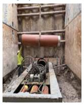
No-Dig Pipe® by Logan Clay Products (Vitrified Clay Jacking Pipe) is predominantly used with the pilot tube method of guided boring for installation of gravity sewers on-grade and on-target at depth and where open-cut is difficult or space is limited. Logan Clay Products 800-848-2141; no-digpipe.com
