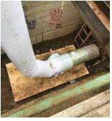
Aegion continues to advance the pipeline rehabilitation market by offering the latest innovations in cured-in-place pipe (CIPP) technology specifically engineered for drinking water applications. The InsituMain™ System, our showcase CIPP innovation for pressure pipe renewal, is a composite material of polyester fiber, fiberglass, and a specially formulated epoxy resin system.
