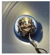
SippTech is revolutionizing pipe rehabilitation with manufactured-inplace composite pipe (MICPTM), MICP is the only robotically installed composite lining system to meet the AWWA Class IV structural/Close Fit Lining (CFL) classification for large-diameter pressure pipes ranging from 48" to 96" with 250+ PSI working pressure capabilities.
