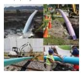
PVC pipe has been in service in North America for 70+ years, with more than 2 million miles installed. It's available in sizes up to 60" for open-cut installations and up to 36" for trenchless applications. PVC pipe has the lowest break rates, lowest environmental
